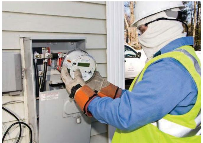
The service entrance was inspected at each meter installation to ensure connections were all good. That is why the installation contractor required installers to wear flash protection.
