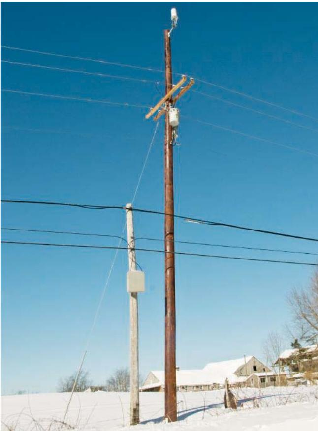
The extender bridge installation on the top of this distribution pole is a typical part of the AMI communications infrastructure.
